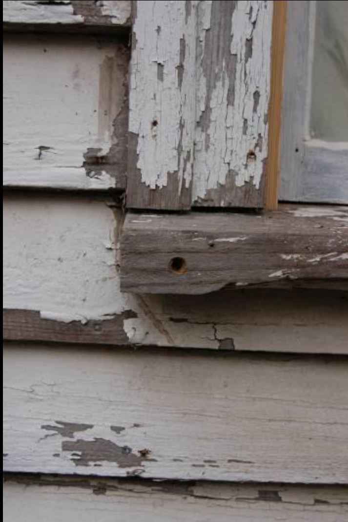
Secure window sills.
