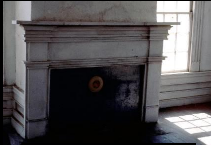
Preserve millwork, including mantels, baseboards, and door and window surrounds.
