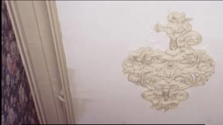
Preserve plaster cornices and centerpieces.
