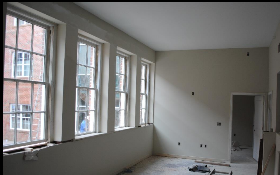
Unit 1D - Later drop ceilings were removed. The volume of space was retained along the exterior wall, but apartments received a one-hour fire rating by installing sheetrock over the plaster walls and wood ceilings and Gypcrete was floated atop the wood floor.
