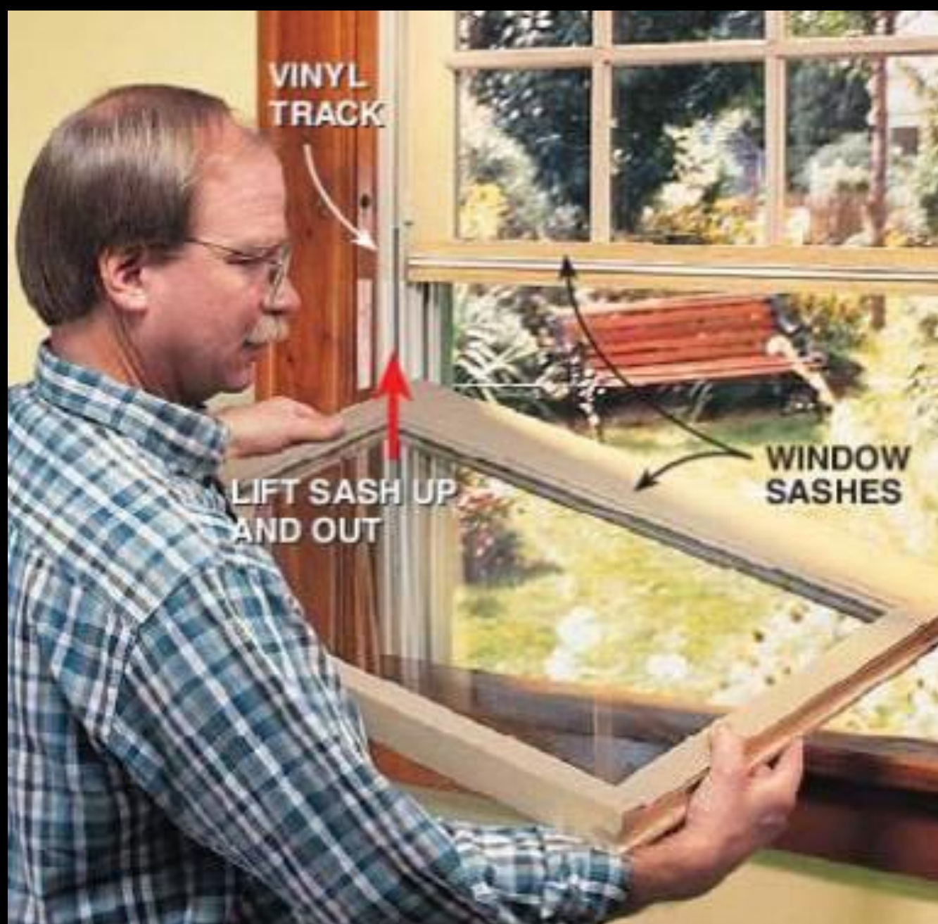
Jamb liners may be needed if sash contain lead paint.
