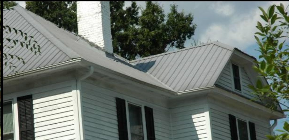
New metal roof. Note large ridge cap.
