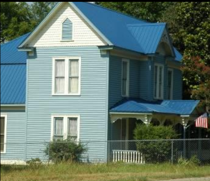
New metal roof. Note large ridge cap.
