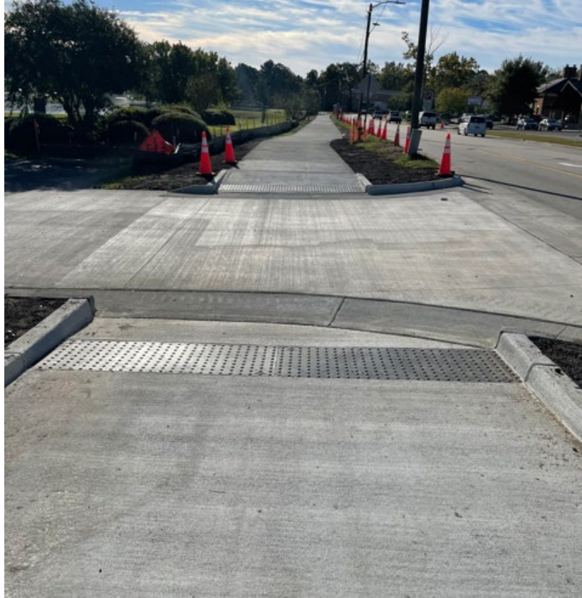
Upgrade of the walking path at the Lake Park to an ADA-compliant multi-use
