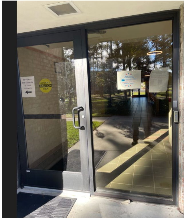
Installation of push-button auto-doors at the rear of Town Hall
