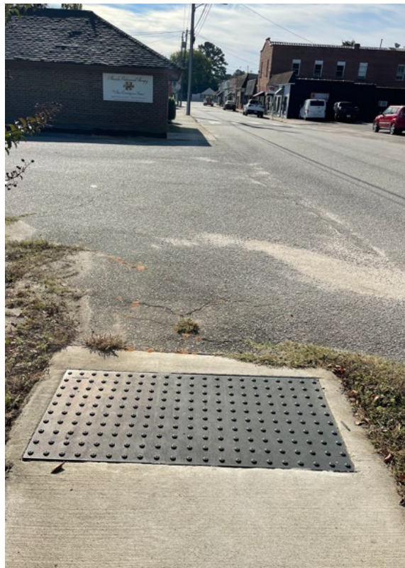
Installation of curb ramps with Detectable Warning Surface on Trade St.
