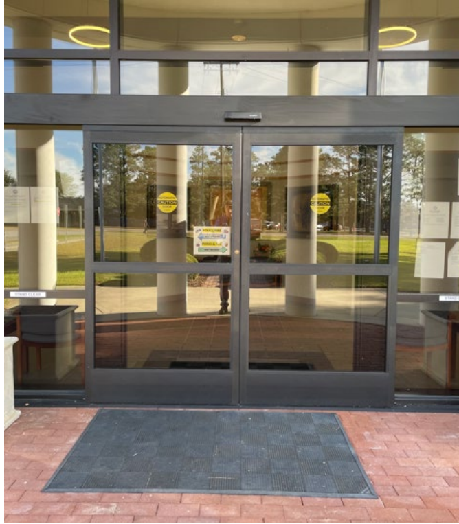
Installation of auto-doors at the front of Town Hall
