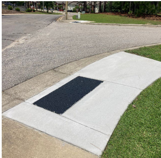
Curb ramps with Detectable Warning Surface on Dunrobin
