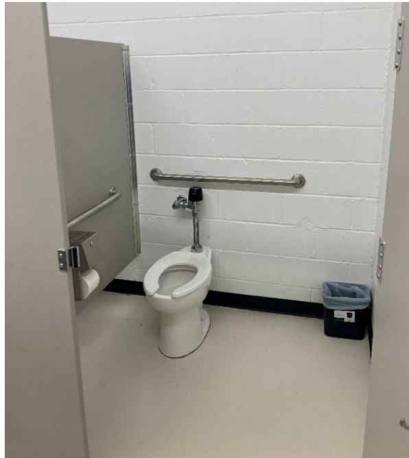
Accessible Restrooms Lake Park Concession
