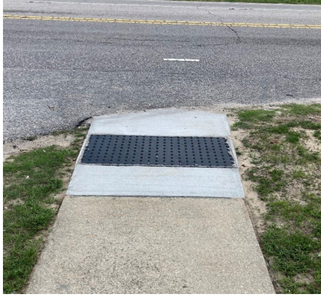
Curb ramps with Detectable Warning Surface at Kensington Village entrance
