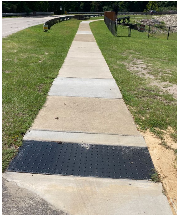
Sidewalk repaired and Detectable Warning Surface installed Lakeview and Lake Shore
