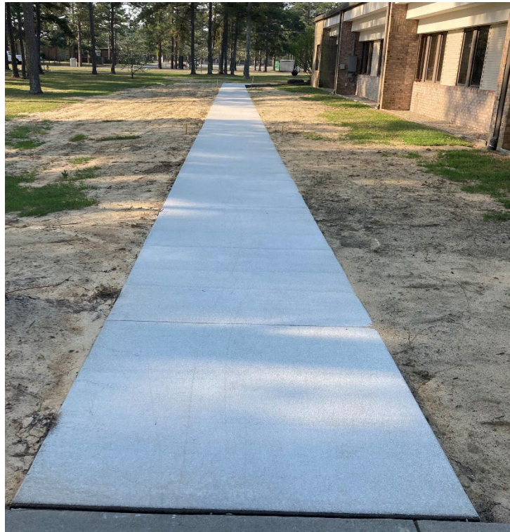
Accessible side walk for access to the front of Town Hall
