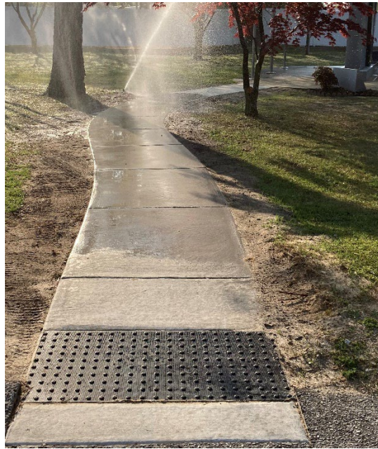
Accessible sidewalk added for access to the Veterans Memorial
