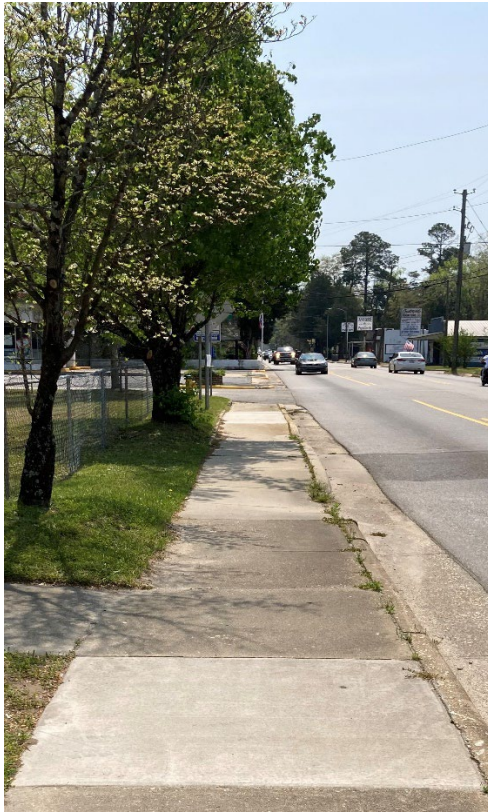
Repairs made to damaged sections of sidewalk along South Main Street
